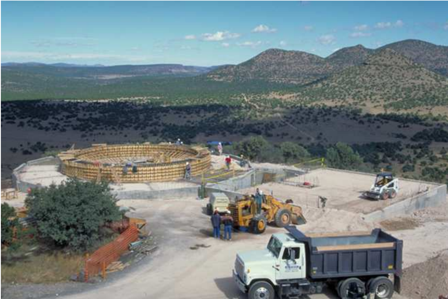
Concrete base, 40 ft diameter, that supports the 9.2m Hobby Eberly Telescope
