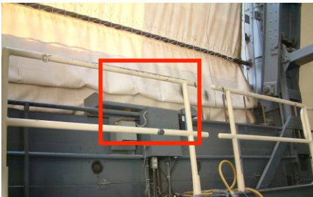
Figure 11: taken by Corby B. Bryan, platform and back up control box above dome rotation point.
