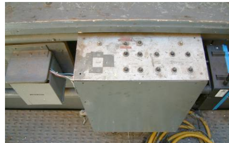
Figure 12: taken by Corby B. Bryan to show backup control of shutters on
