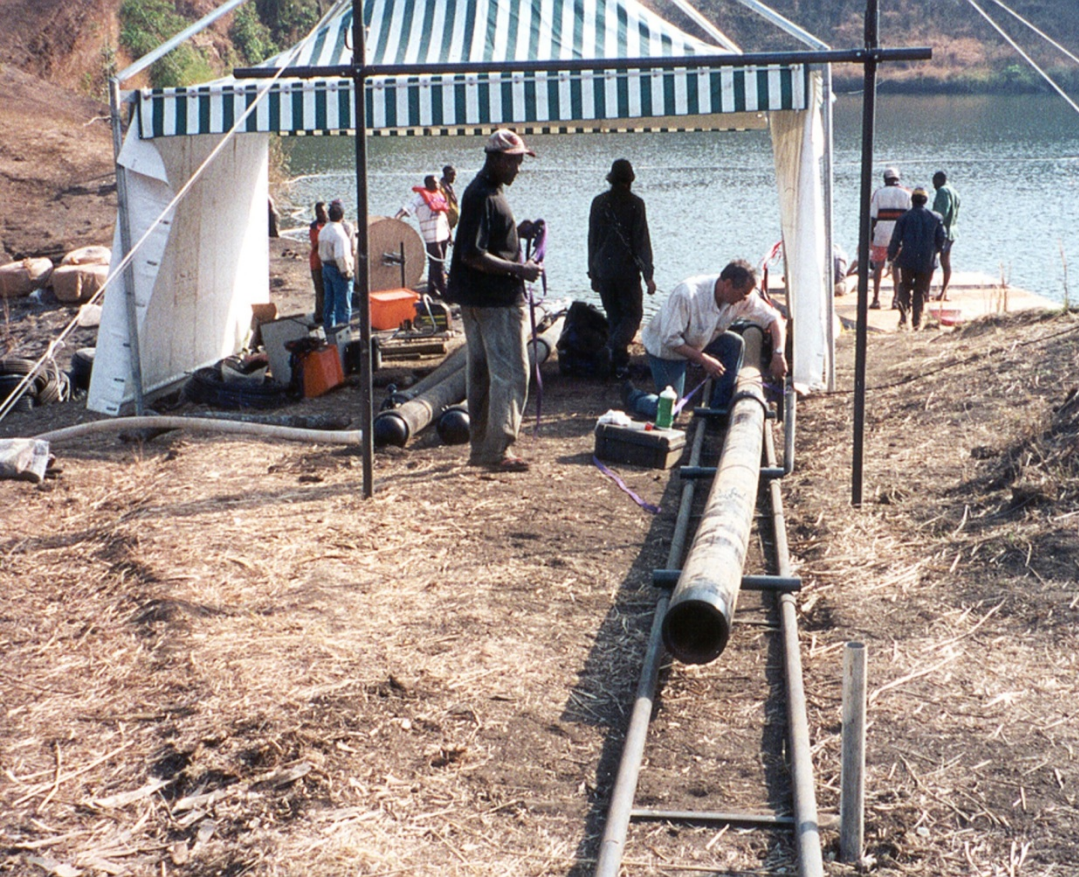
French engineers led by Michel Halbwachs oversee pipe assembly on the shore of Lake Nyos.
