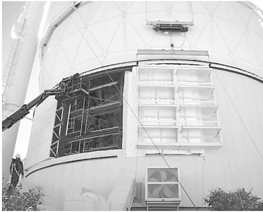
Figure 5: Louver crane in operation, preparing to install second louver module in the north side of the ring wall.
