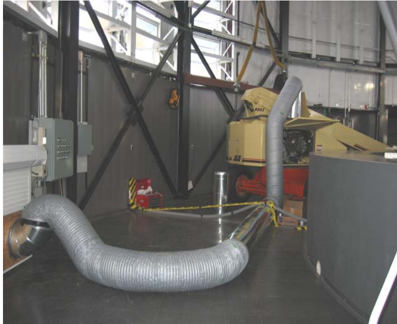
Figure 7: Early operation of JLG ducting
